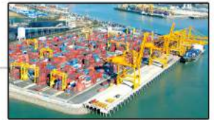
Incheon container terminal
